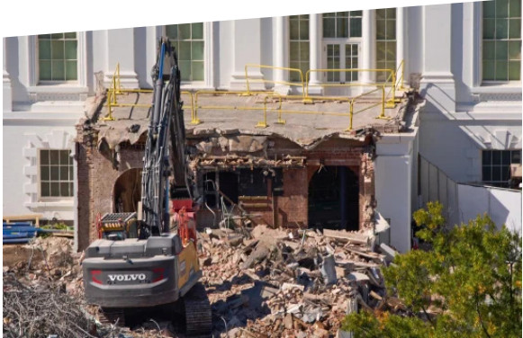
Before and After: The White House’s East Wing gets demolished. Photo courtesies of ABC.
